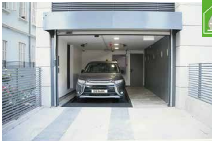
Transfer cabin with concrete walls and roof
