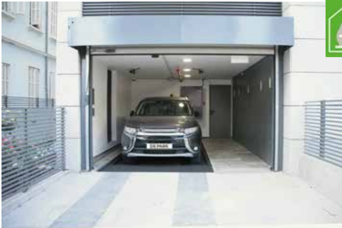
Transfer cabin with concrete walls and roof
