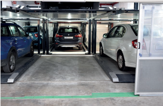
Figure above: DE-611 system for demonstration only.
